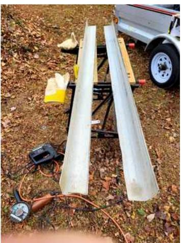
These are post supports for Marion's North fence. It started off as a square extrusion and has been cut into two right angle girders. These are to be concreted into the ground and the shortened fence posts connected to them above the soil. A sterling effort by all those involved especially with the onset of Winter.
